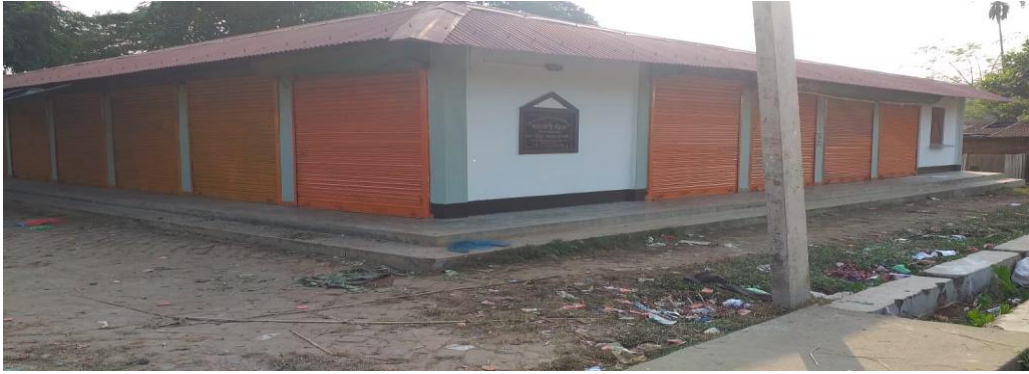
Maket Stall Constructed From SC Welfare DEPT
