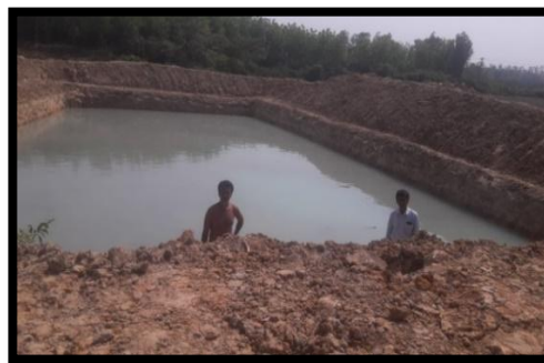
Construction on new pond
