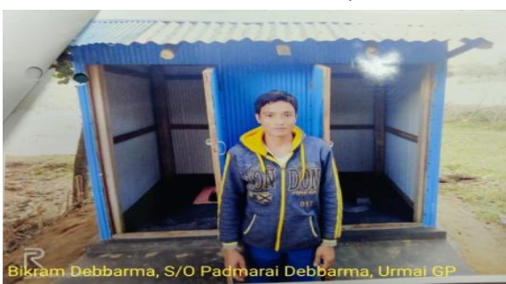
Twin leach pit toilet constructed under SBM-G Scheme
