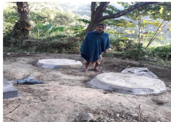
Twin leach pit toilet constructed under SBM-G Scheme
