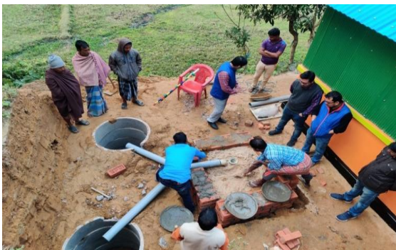
Ongoing construction of twin leach pit toilet under SBM-G
